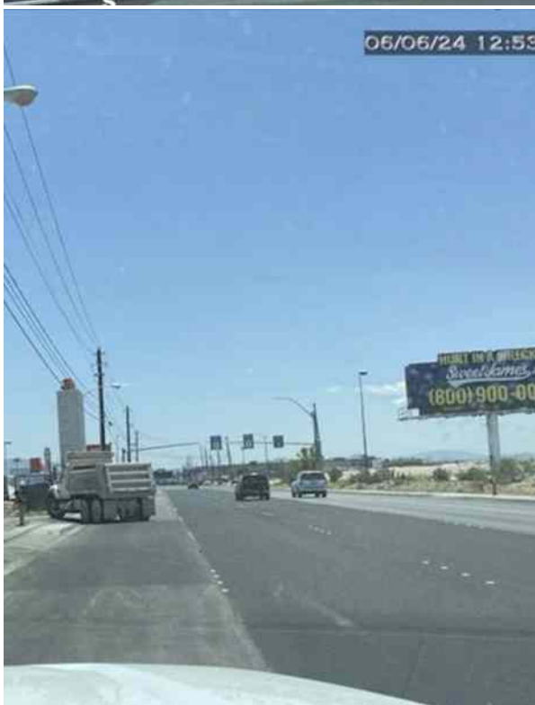
Photos taken by a Clark County official show a truck hauling waste from a Boring Company worksite on June 6, 2024. The official observed mud spilling from the vehicle. The photos were obtained through a public records request. (Credit: Clark County Road Division)
